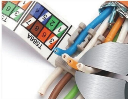
5. Cut the extra cables from the cap.
