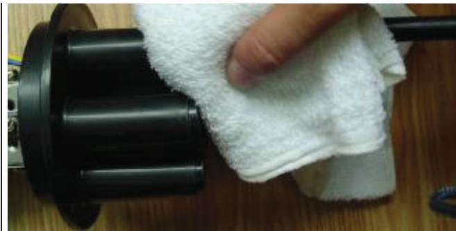
(10)Sealing of cable and base: clean the entry ports and cable for 10cm with alcohol
