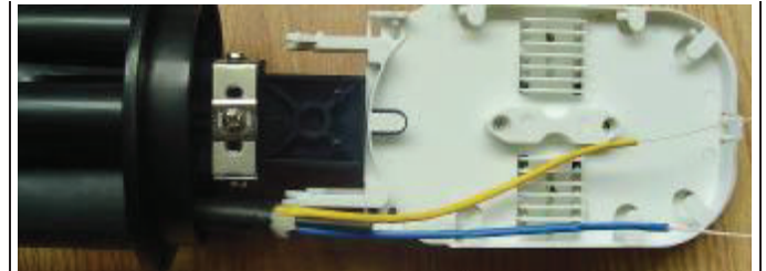
(3) push the cable onto the bracket through the entry ports.
